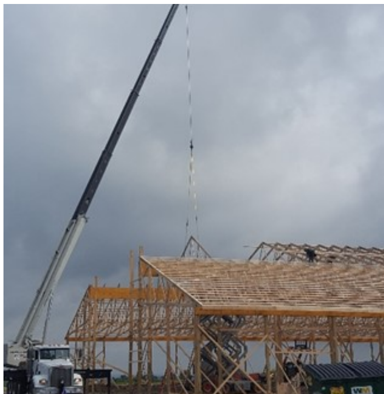
Pictured: Roof trusses being installed on the new dairy barn.
