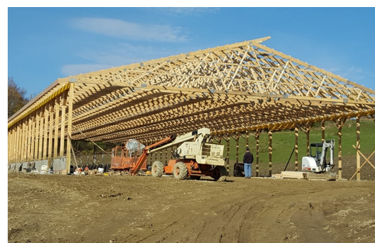
Figure 1— Initial Framing for new robotic milking barn. Canaseraga, NY (Allegany Co.)
