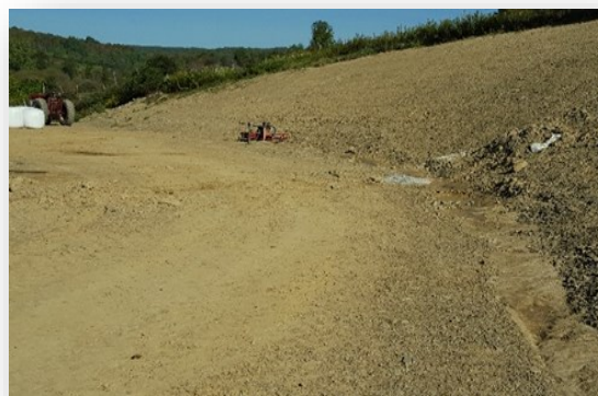
Graded and shaped diversion ditch around beef facility ready for seeding and mulching.
