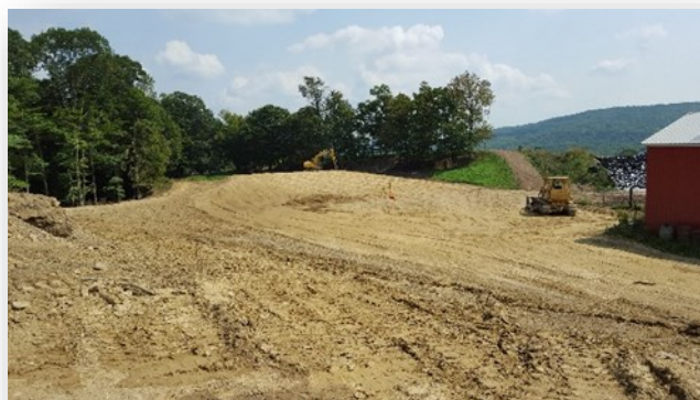
Graded pad for new heifer & dry cow barn near Canaseraga, NY (Allegany Co.)
