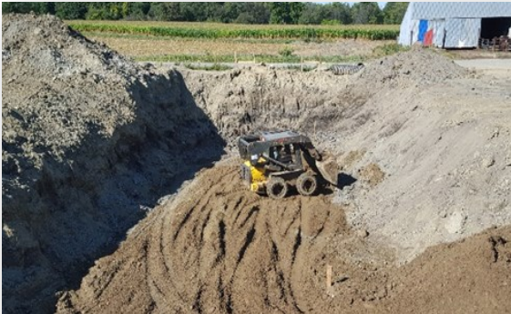
Gravel subgrade going in for an ag waste storage tank in a new milking center. Bliss, NY (Wyoming Co.)
