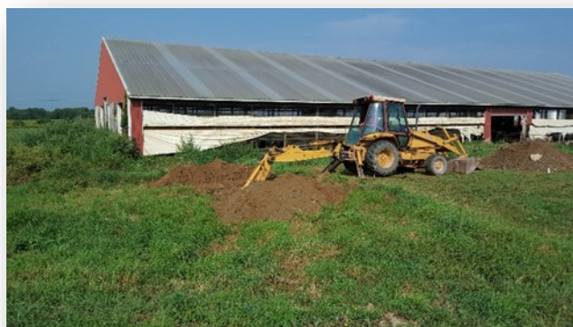
Test pits being dug for an ag waste storage south of Avon, NY (Livingston Co.)
